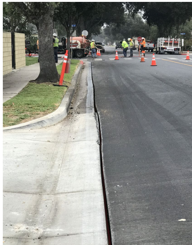
Figure 3: Microtrenching work in progress in Fullerton, CA. Photo by Fullerton Observer.
