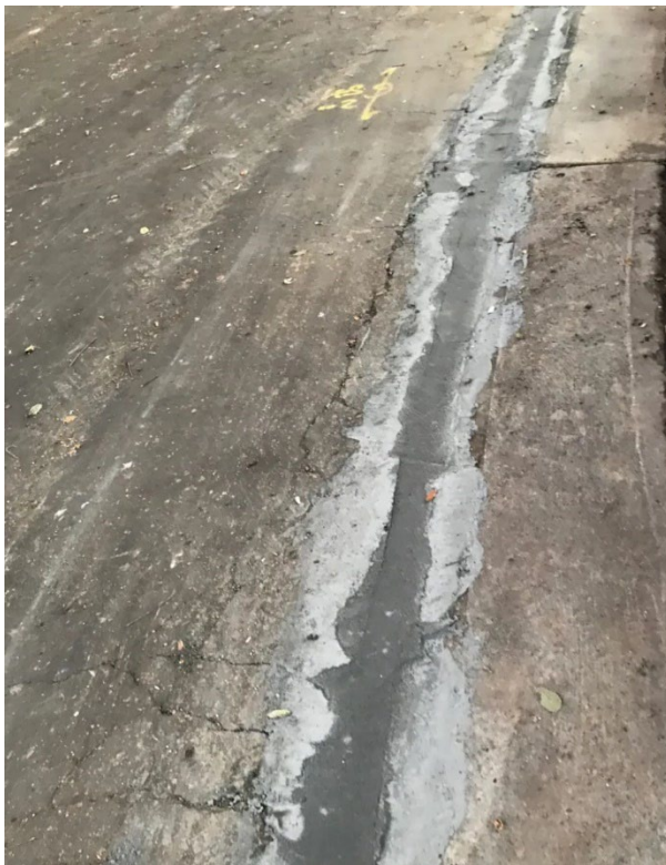
Figure 2: Microtrenching work completed in Fullerton, CA. Photo by Fullerton Observer.
